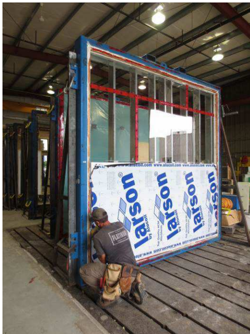
Figure B2 – Lower Panel Installation
